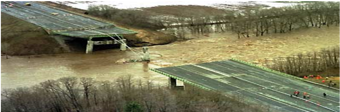
Figure 1.1: Extreme events, such as floods, can result in severe infrastructure damage, bridge collapse. A capable Autonomous Surface Vehicle (ASV) can assess the soundness of the structure in a safe and timely manner.
